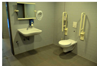
Douche/wc in de kleedcabine
